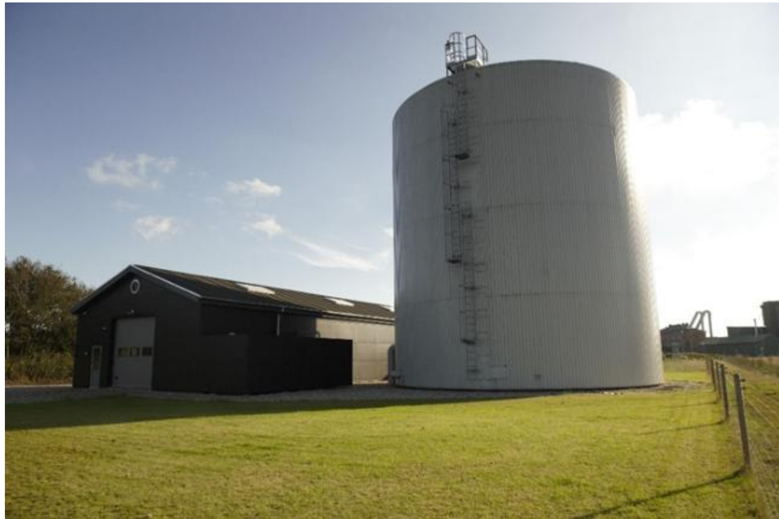
TTES à Karup (Danemark) – 3'600 m 3 . Photo: Karup district heating
